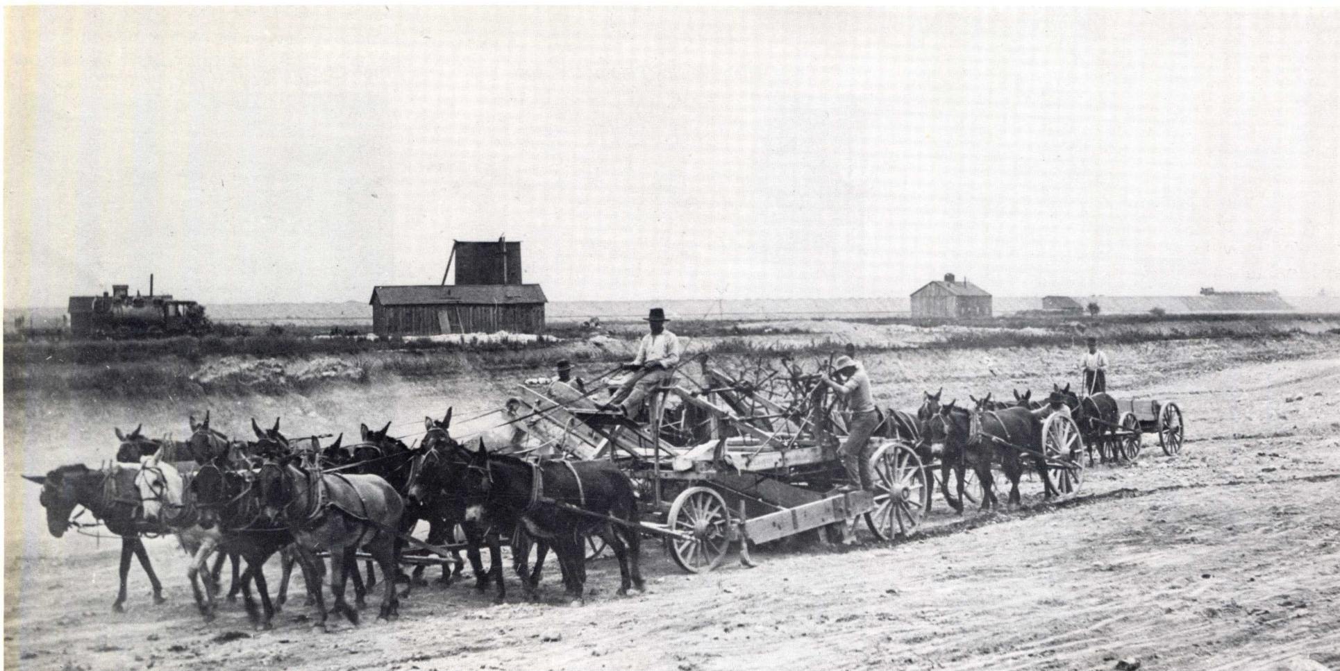
A mule-drawn grader preparing the canal bed in 1894 for the Chicago Sanitary and Ship Canal. Opened in 1900 the canal supplanted the function of the Illinois-Michigan Canal of 1848.
