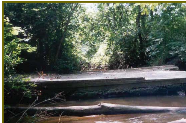
Problem Hydraulic Structure (fallen bridge) in Reach BC13
